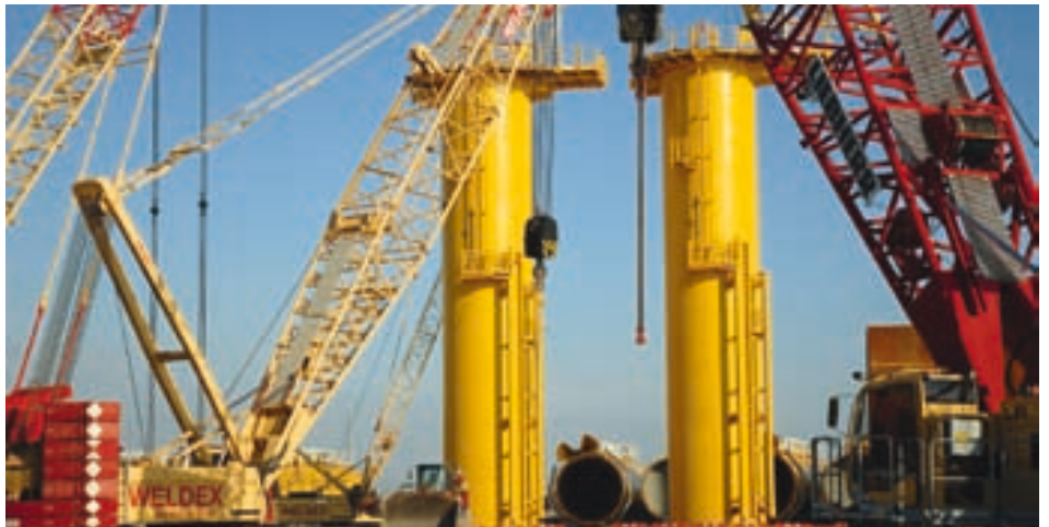
Port side construction work for Rhyl Flats Offshore Wind Farm
